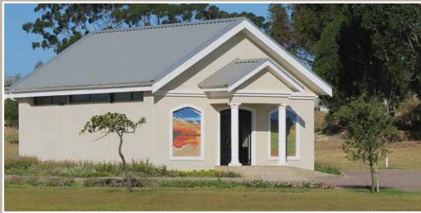
Columbarium Building provides indoor above ground ash niches.
